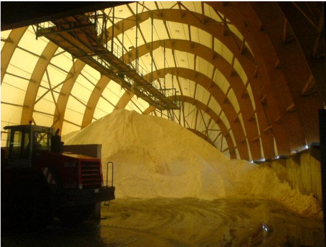
Figure 1: Salt storage of DEUSA International GmbH
