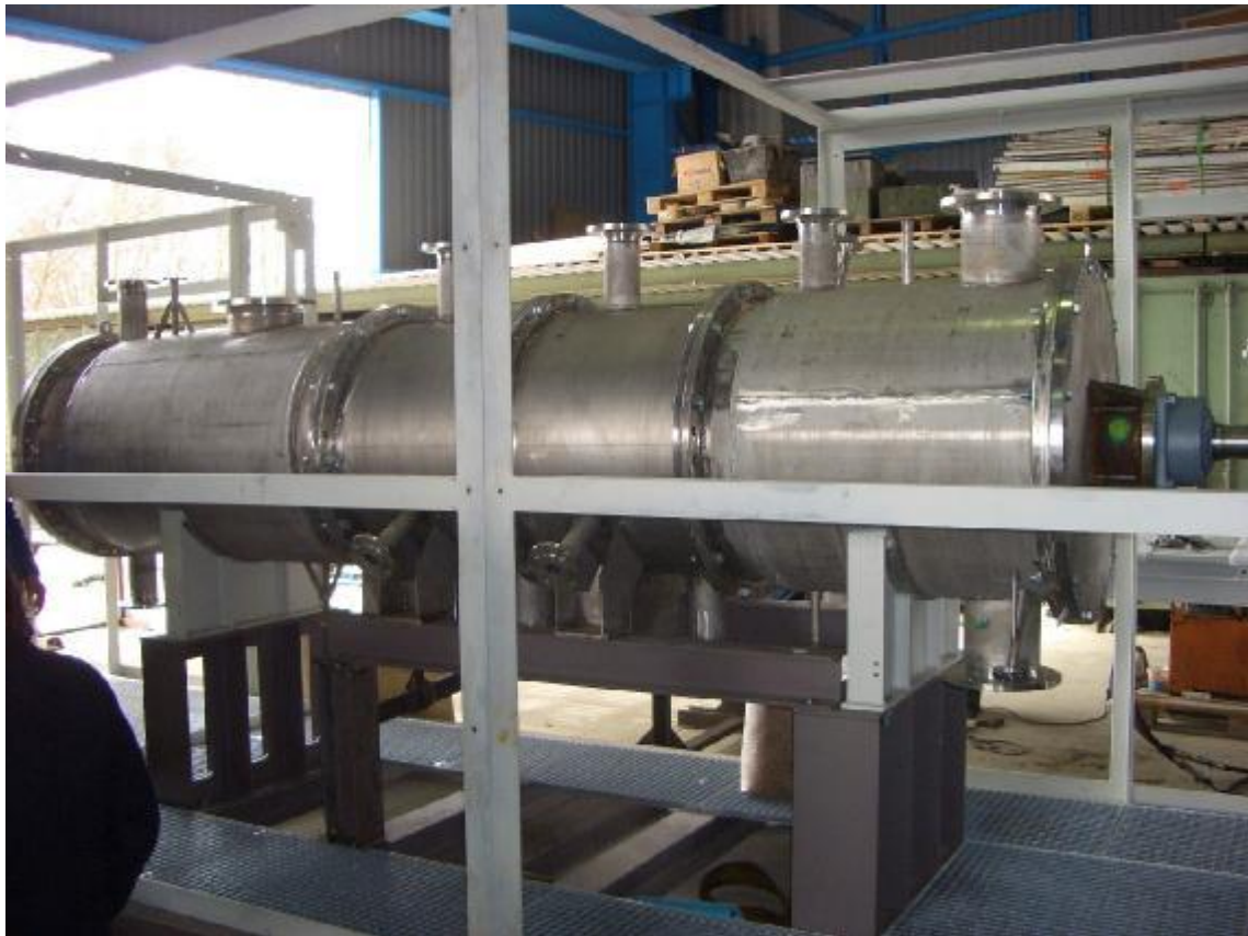
Picture 2: Module 1 to 4 – installation of LMSV
